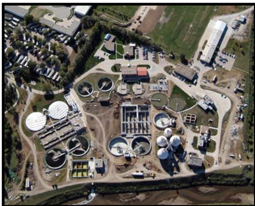
Theresa Street WWTP
