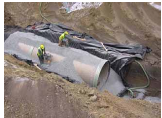
Backfill operations on 84-inch diameter pipe
