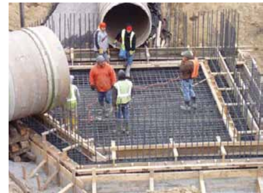
Junction Structure near Northeast Treatment Facility – 84-inch diameter & 60-inch diameter pipe
