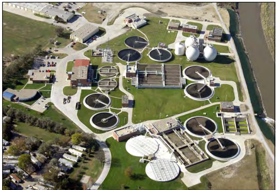
Theresa Street Treatment Facility
