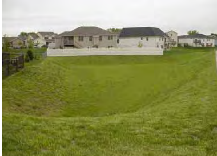
Dry Detention Basin at NW 12th St & Keating Drive,
