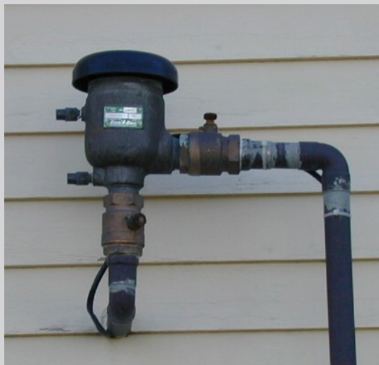
Typical backflow device for a lawn irrigation system.
