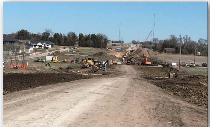
*Grading and stormwater drainage work on Rokeby Road looking east from S. 74th Street*
