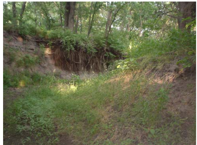
Type IV stream reach located upstream of SW 12 th Street
