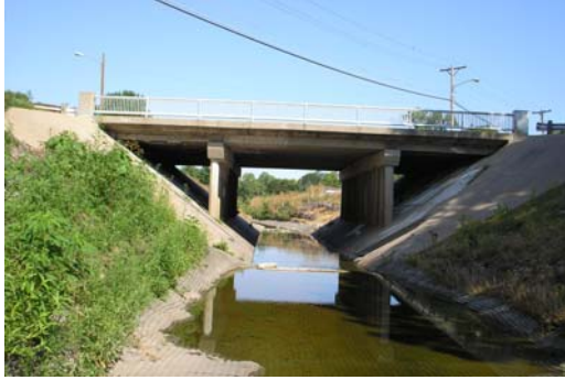
52 nd and Francis Street Bridge Crossing
