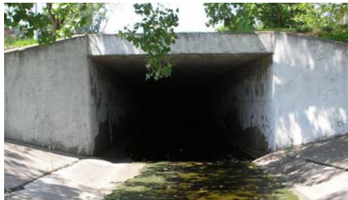
Culvert extending beneath MoPac Trail just north of "O" Street
