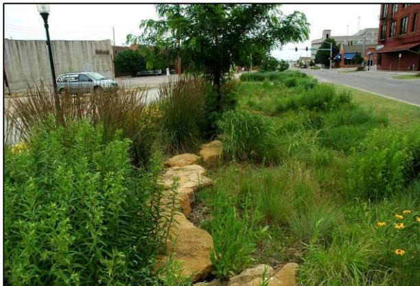
Example of bioretention cell
