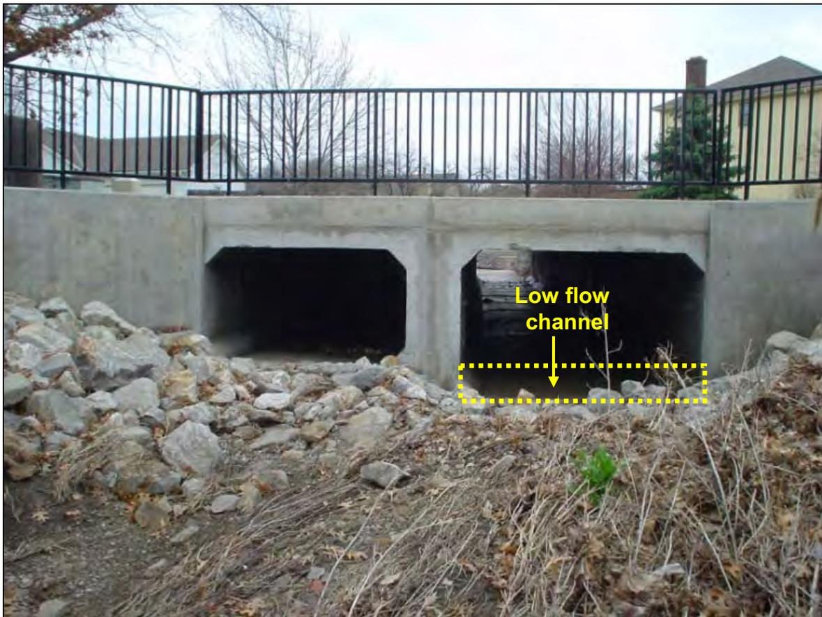
**Figure 7-1: Conservation culvert example**
