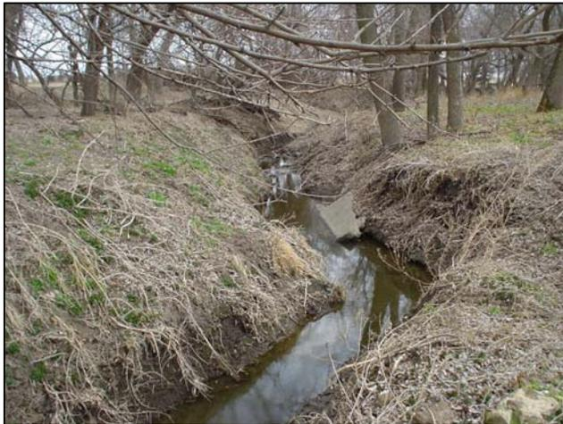
**Figure 8-3: Incised V-shaped channel on Tributary 220**
