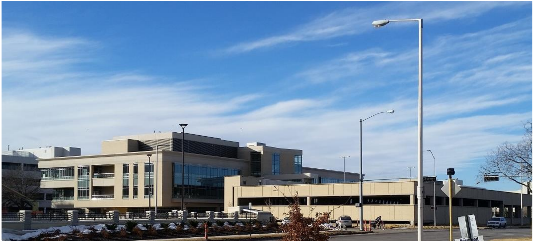
▲ III Landmark Centre from northeast
