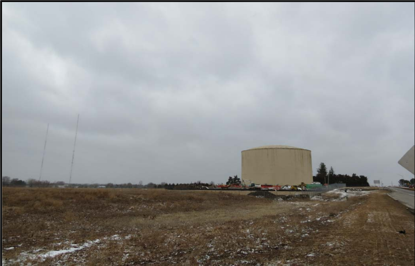
1 LOOKING NORTH-WEST BEFORE SCALE: N.T.S.
