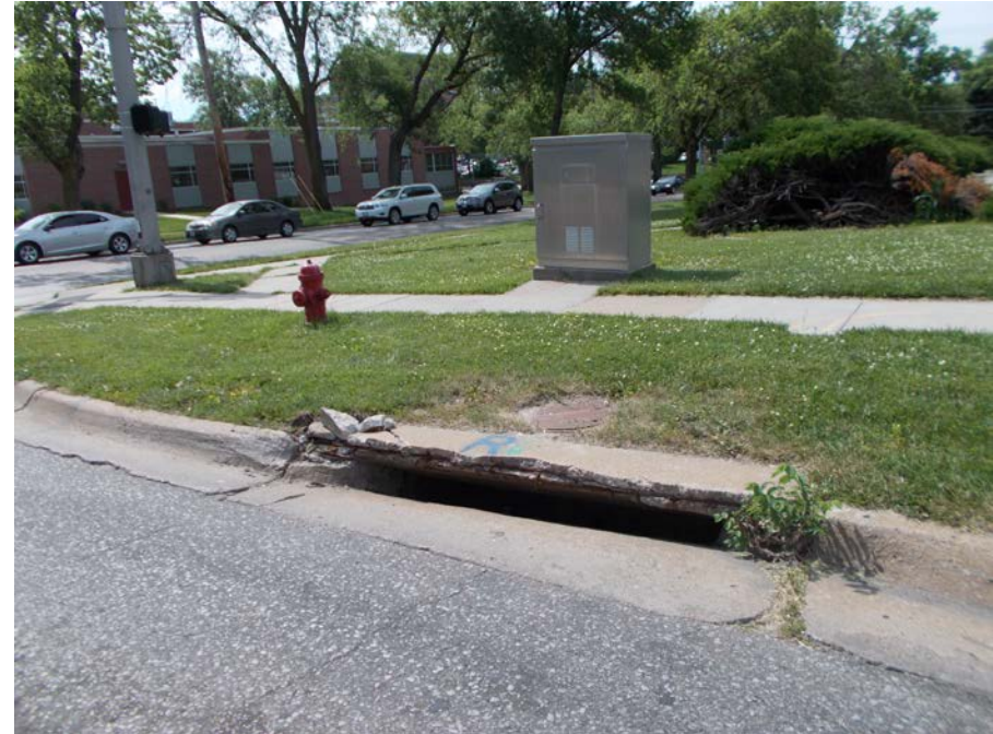
Damaged storm inlet top
