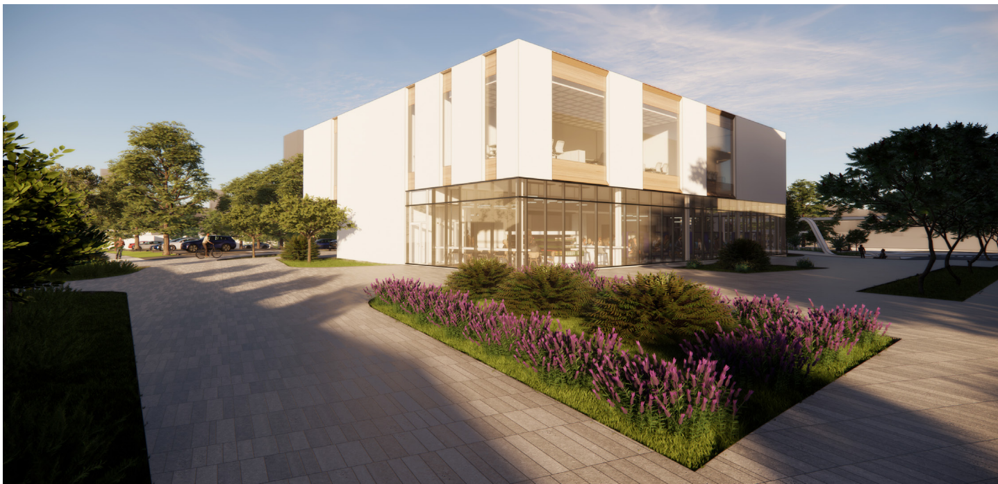
View of MMTC from the preferred location near 10th & H streets looking southwest
