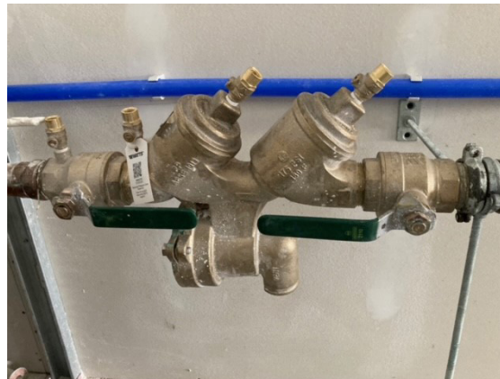
Example of a backflow device that can be used on a swimming pool and/or boiler.
