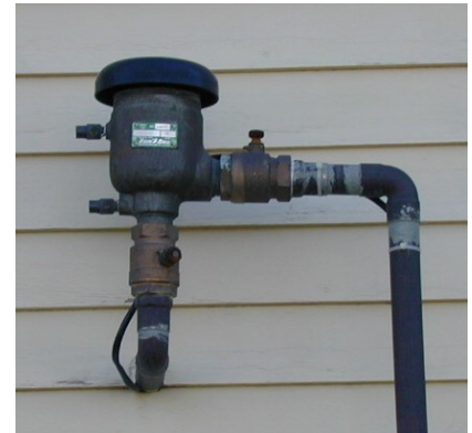
Typical backflow device for a lawn irrigation system.
