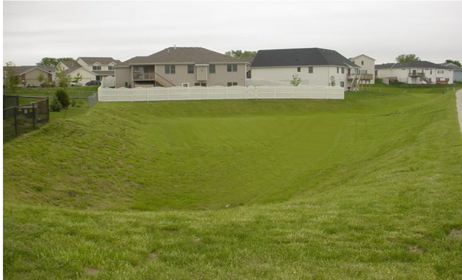
Detention basin located at NW 12th Street & Keating Drive, Lincoln, NE
