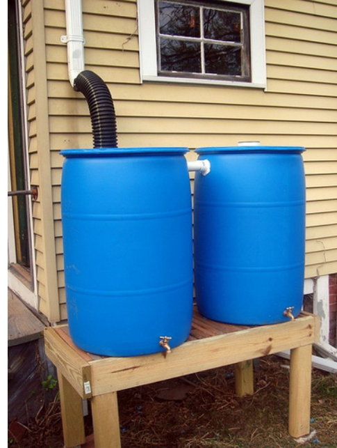
Rain barrels installed on residential properties
