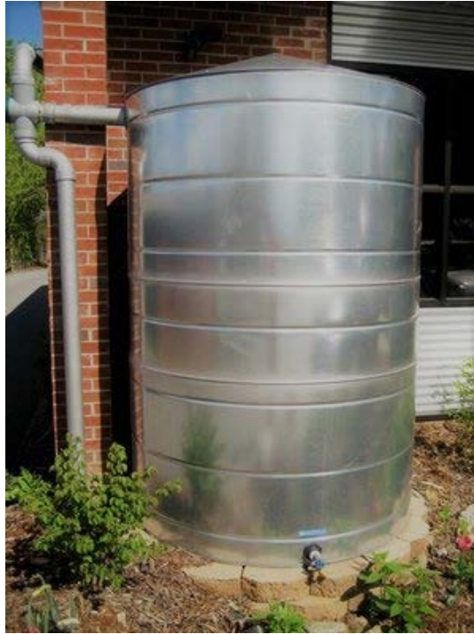
Larger rain barrel installed on commercial property Source: Higher Ground Rainwater Systems
