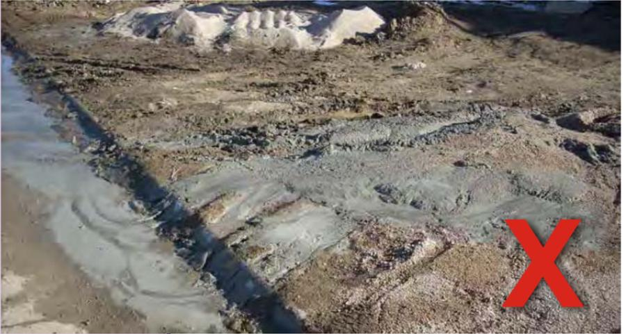
Each development should have designated concrete washout areas. If none exist contact the developer. The photo below is one example of a concrete washout area. There are many variations and designs for concrete washout areas. If maintenance is needed contact the developer. Never wash concrete into the storm drain.
