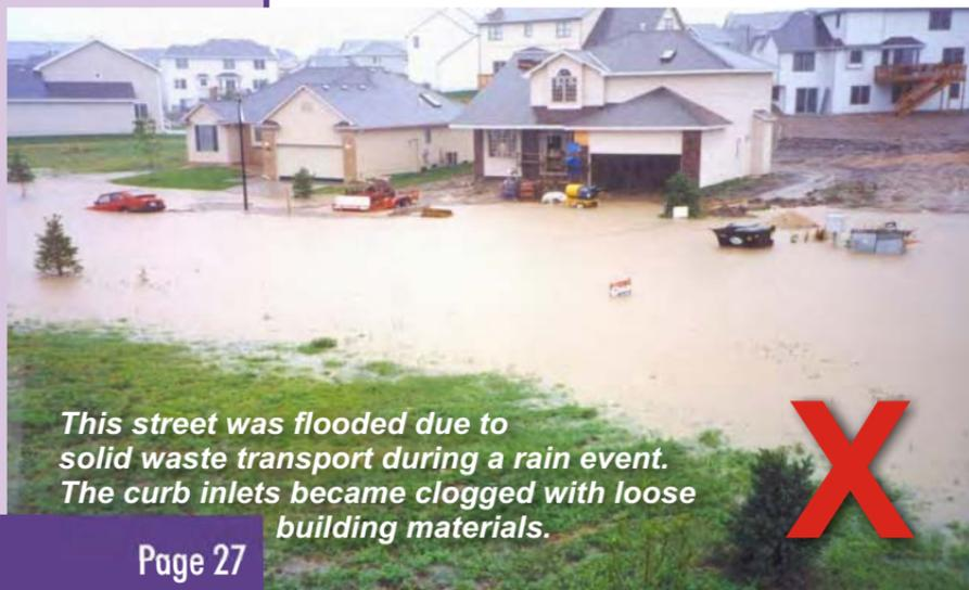
*This street was flooded due to solid waste transport during a rain event. The curb inlets became clogged with loose building materials.*
