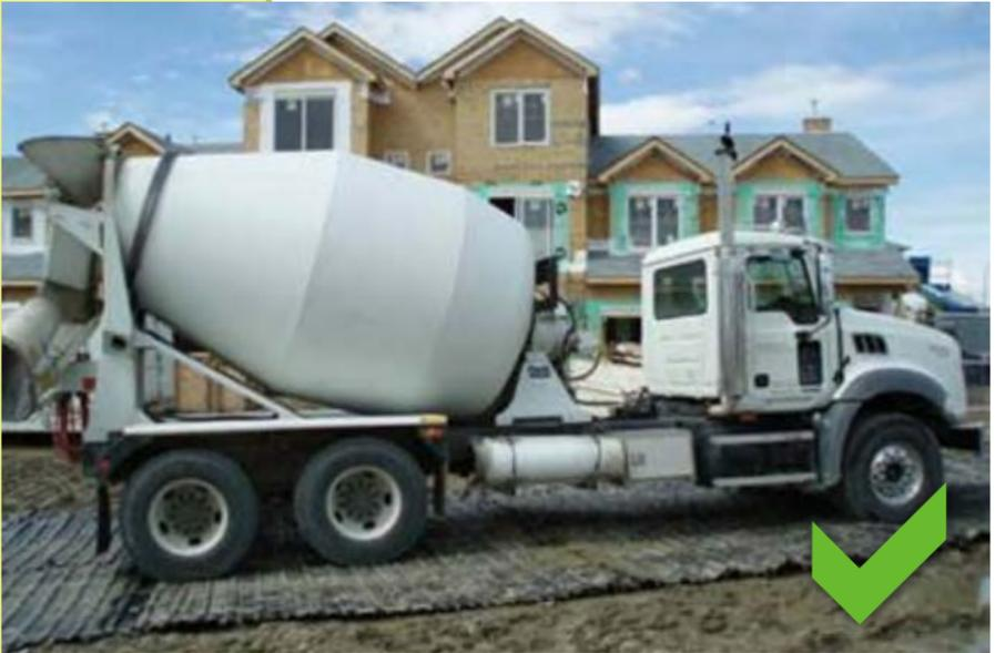
The above picture shows the use of vehicle tracking pad. Even in wet conditions there is no mud tracking.
