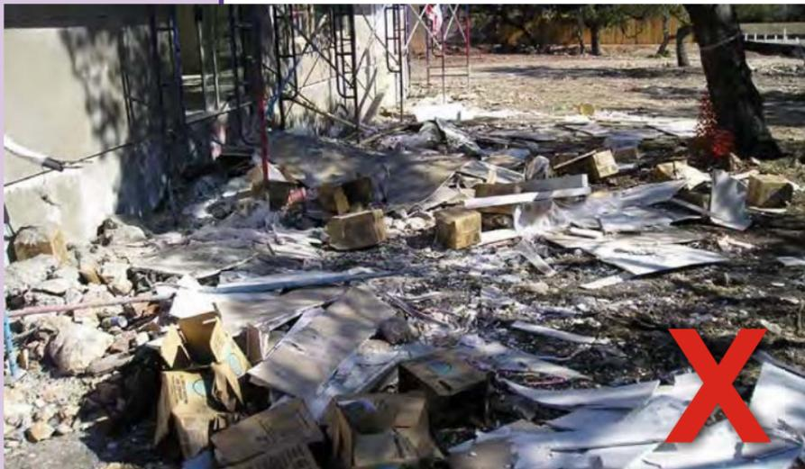
This is a combination of scrap drywall, drywall compound slurry, and other solid waste. The drywall slurry is considered a chemical spill, which is a violation.
