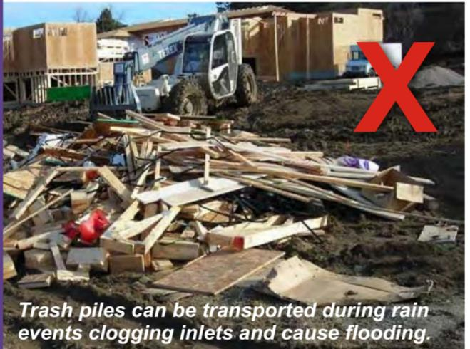
*Trash piles can be transported during rain events clogging inlets and cause flooding.*
