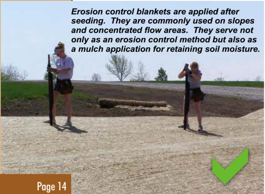
*Erosion control blankets are applied after seeding. They are commonly used on slopes and concentrated flow areas. They serve not only as an erosion control method but also as a mulch application for retaining soil moisture.*
