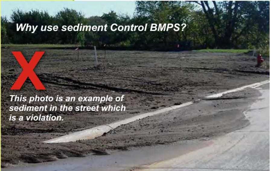
Once vegetation has been stripped from the home site, sediment controls to protect the public right-of-way are the only option. Sediment control BMPS will not only help reduce sediment in the right-of-way, but will also assist in minimizing track out.
