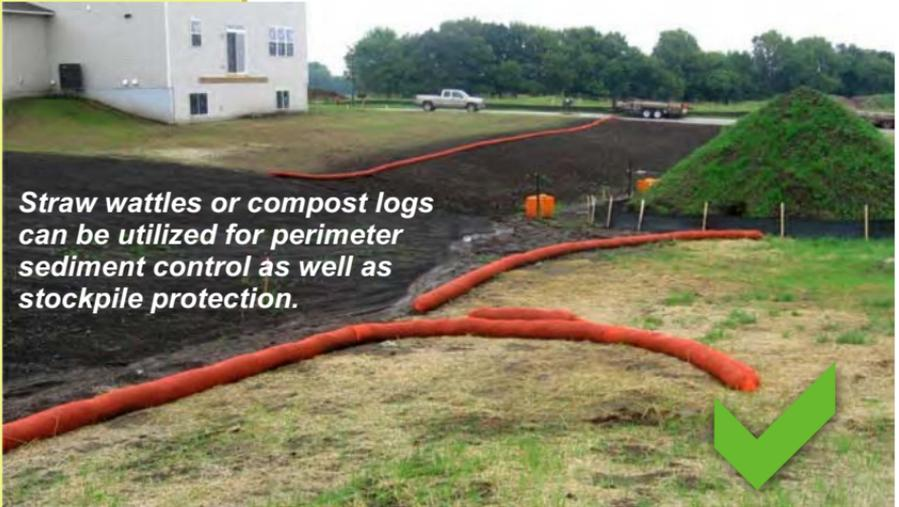
**Straw wattles or compost logs can be utilized for perimeter sediment control as well as stockpile protection.**
