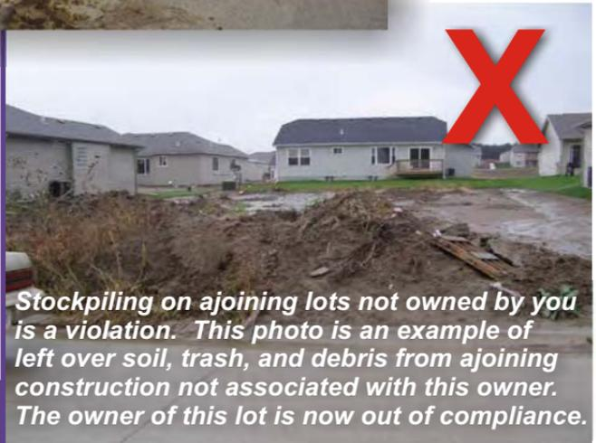
*Stockpiling on adjoining lots not owned by you is a violation. This photo is an example of left over soil, trash, and debris from adjoining construction not associated with this owner. The owner of this lot is now out of compliance.*
