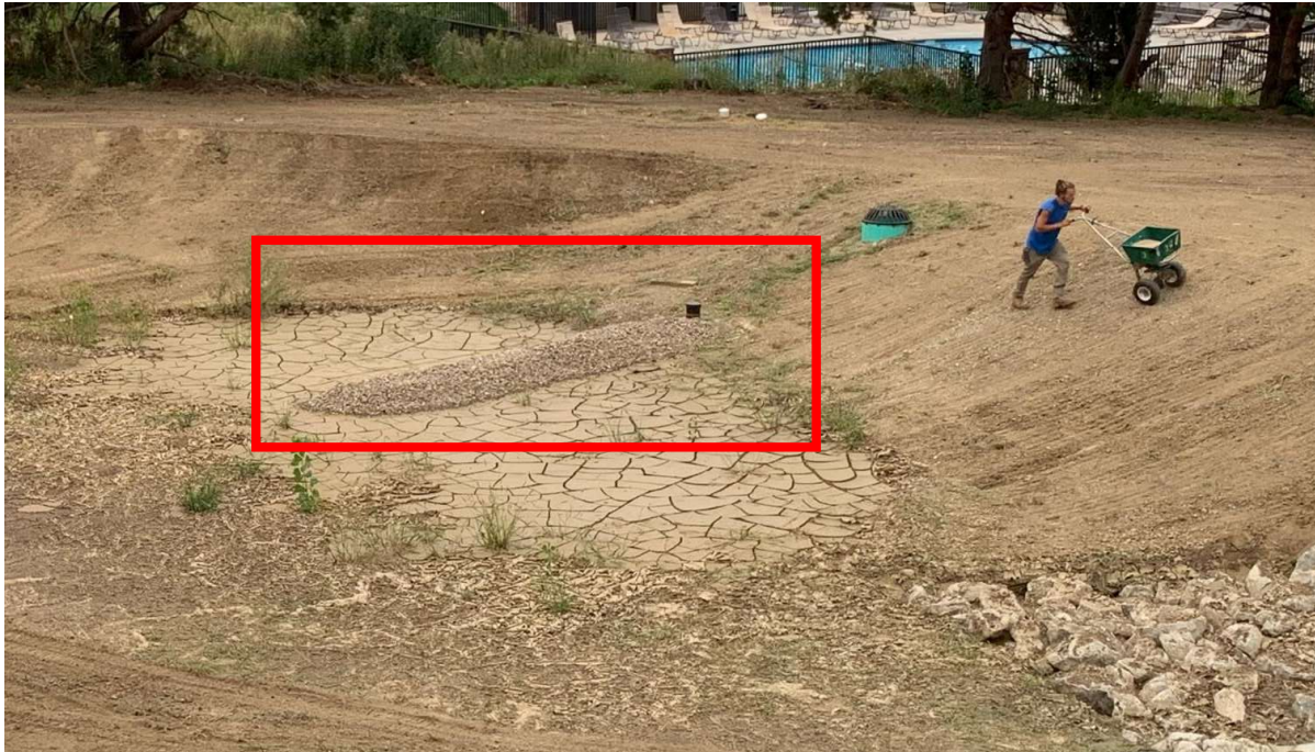
Horizontal Underdrain with rock filter
