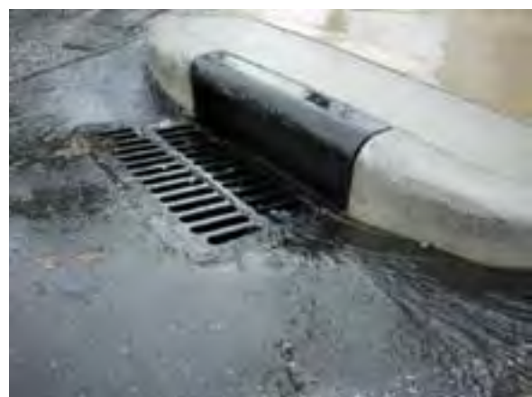
Stormwater Services of Wilmington, NC
