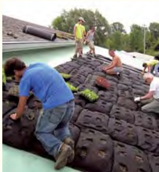
Milwaukee Metropolitan Sewerage District
