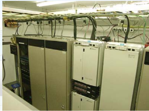
New beside old: Twice as many paths, quadruple the capacity. Same footprint. 10 years newer. That's microwave technology.
