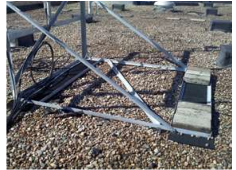
Non-penetrating roof mount antenna system at new EOC facility
