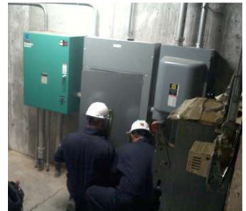
Contractors in arc-flash suits examining moisture related failures in high-voltage 911 feeder circuit.
