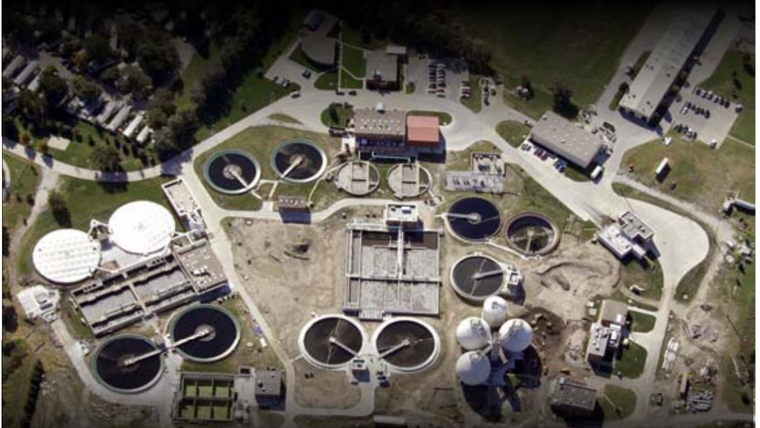
Theresa Street Treatment Plant
