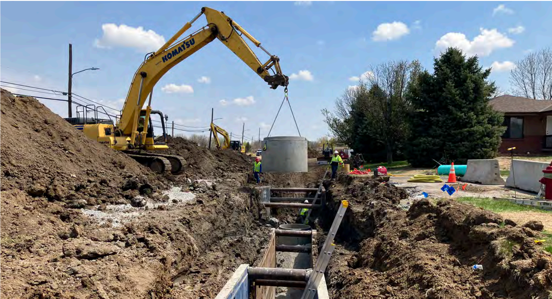
Installed manhole with backfill
