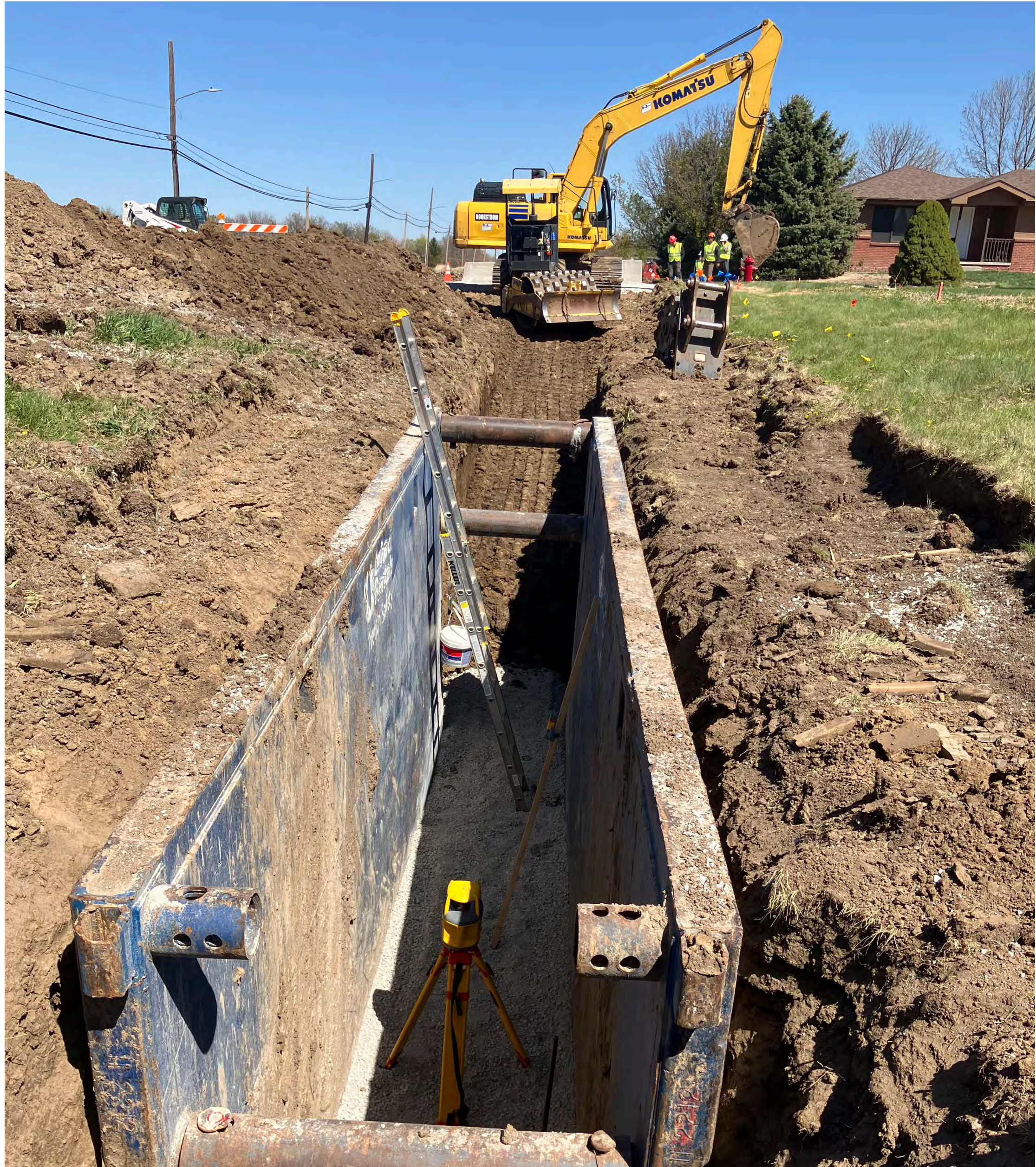
Surveying pipe alignment
