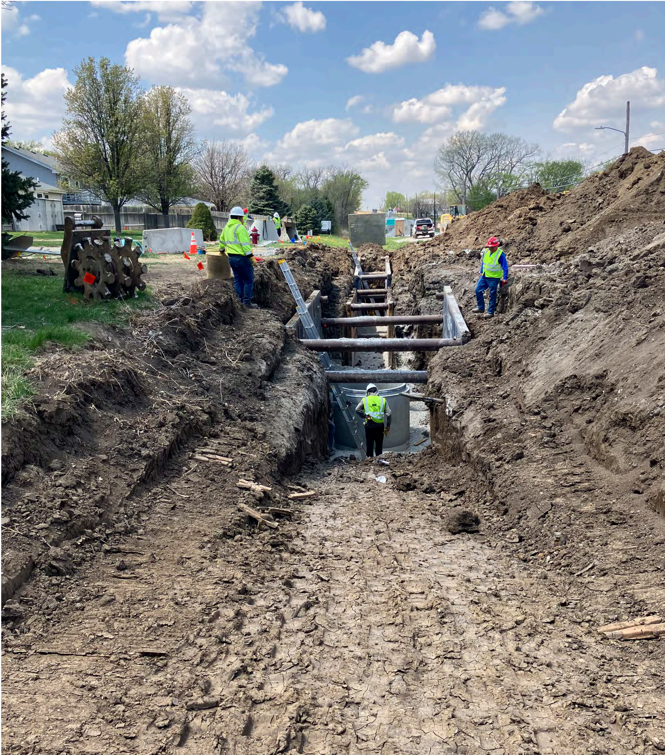
Installing a manhole
