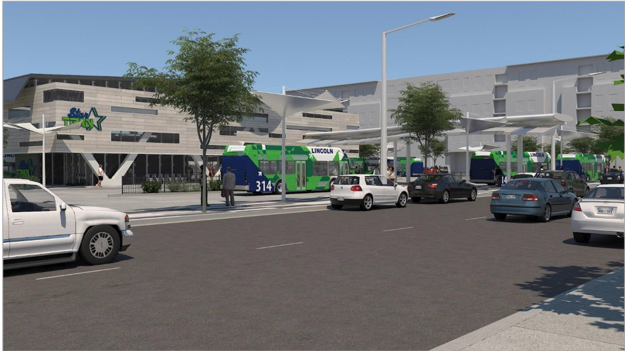
Figure 60: MTTC Concept - View 2 (Looking from M Street and 9th Street to the Northeast)
