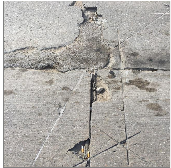
Saw-cut Loop Wire Damage
