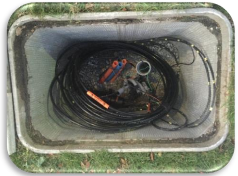
Fiber Box with Splice Enclosure
