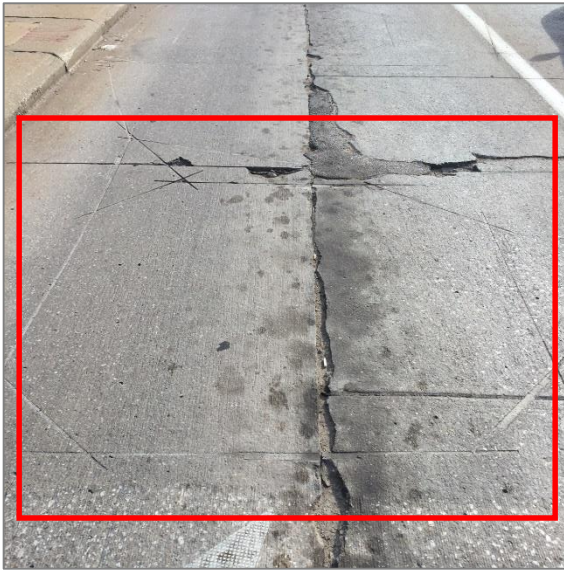
Saw-cut Loop in Damaged Pavement
