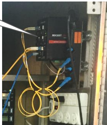
Switch with Fiber Jumpers
