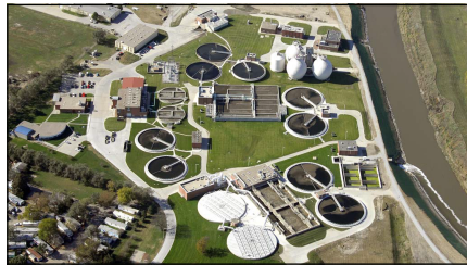
Theresa Street Water Resource Recovery Facility
