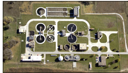
Northeast Water Resource Recovery Facility
