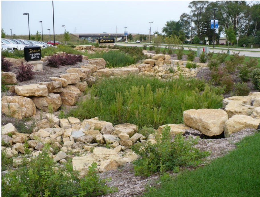
Infiltration Basin utilizing native plants and decorative boulders
