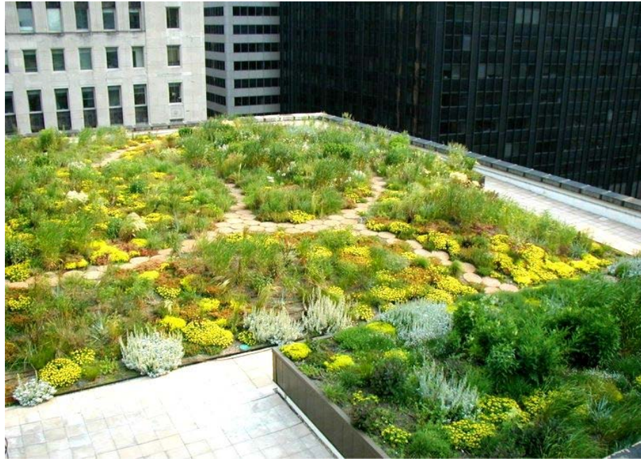
Chicago City Hall, Chicago, Illinois source: greenroofs.com
