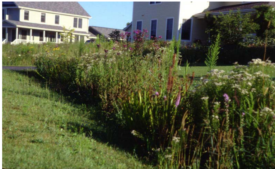
Bioswale using native plantings in a residential applicable
