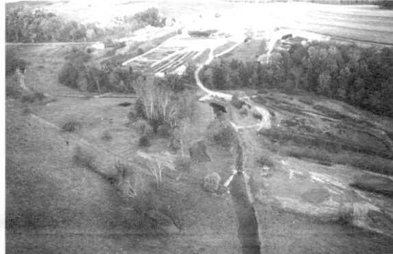
Octoraro Creek, Lancaster County
