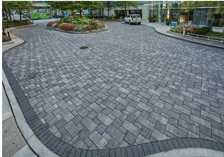
Decorative permeable paving system installed in public square
