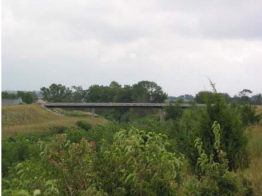
Photo 36. Oak - US face of airport bridge
