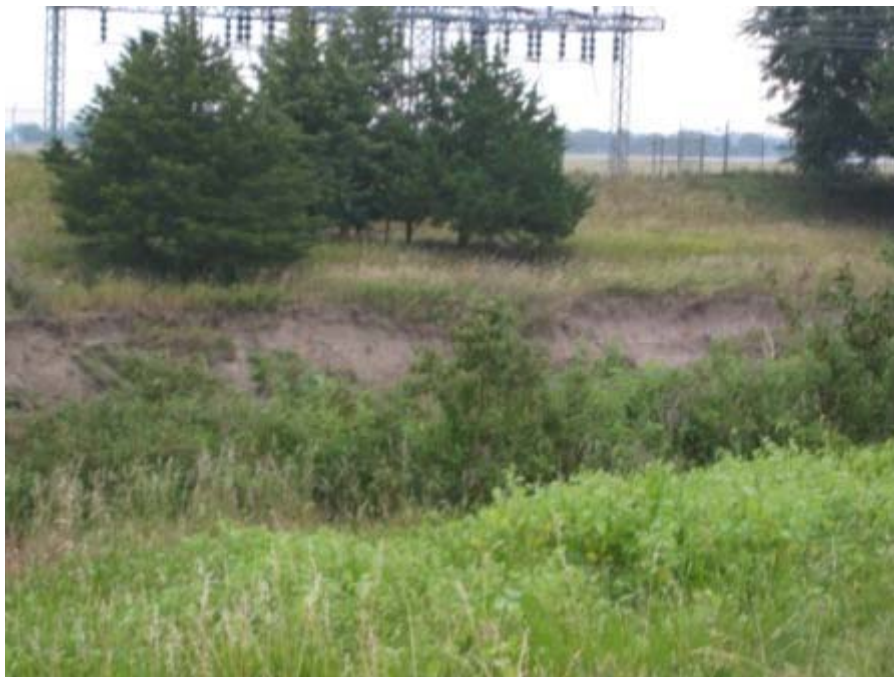
Photo 33. Oak - Substations from RB
