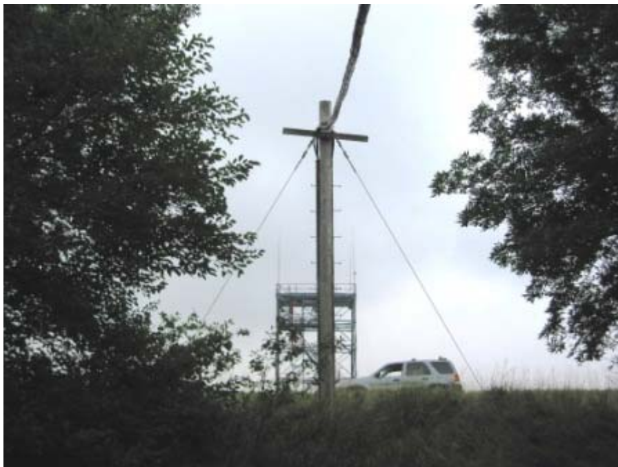
Photo 19. Oak - Communication line and abandoned radar tower from Oak RB
