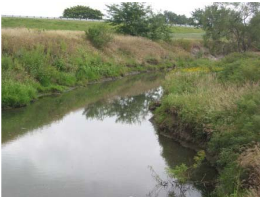
Photo 23. Oak - Looking DS from Air Force Base local drainage culverts
