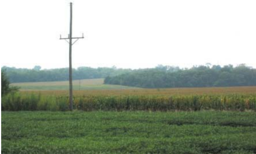
Photo 26. Oak - Power line towers - front tower part of known alignment, rear towers part of unidentified alignment
