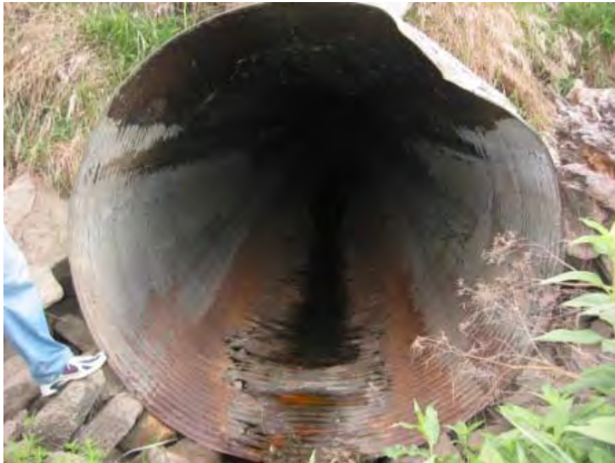
Photo 15. Oak - Air Force Base local drainage culverts US face at levee road - one barrel
