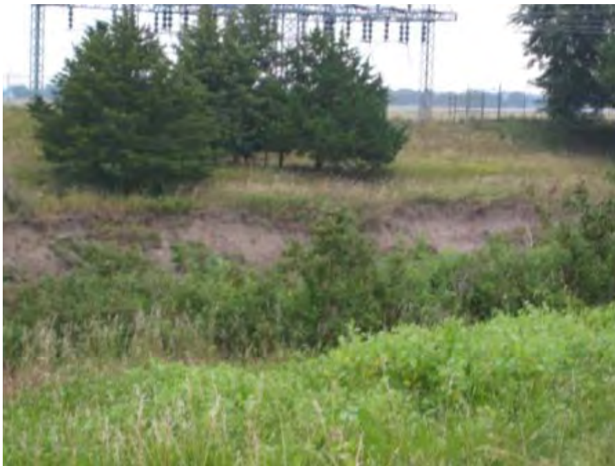
Photo 33. Oak - Substations from RB
