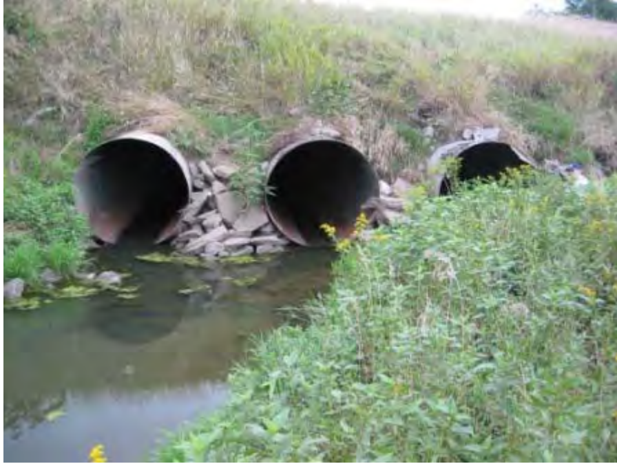
Photo 14. Oak Site - Air Force Base local drainage culverts US face at levee road
