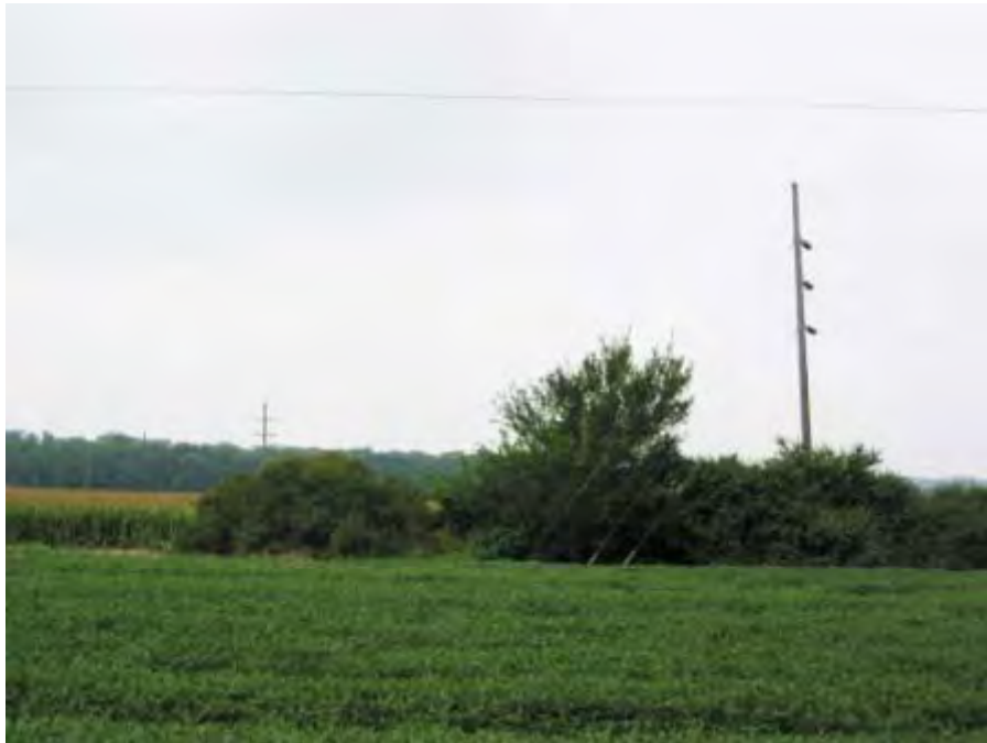
Photo 28. Oak - Small unidentified power line from RB looking southwest
