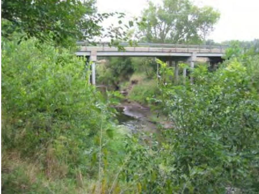
Photo 5. Middle Site - DS face of SW 40th St. bridge
