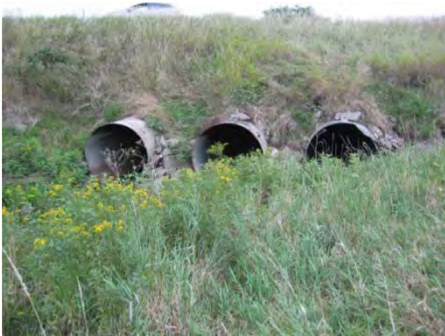
Photo 16. Oak - Air Force Base local drainage culverts US face at levee road
