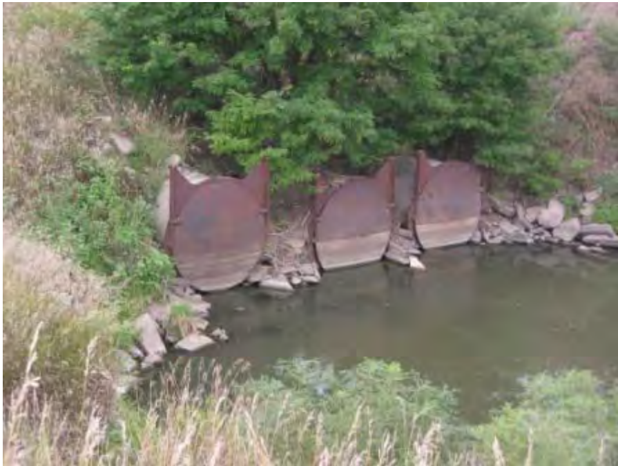
Photo 17. Oak - Gates on Air Force Base local drainage culvert outlets
