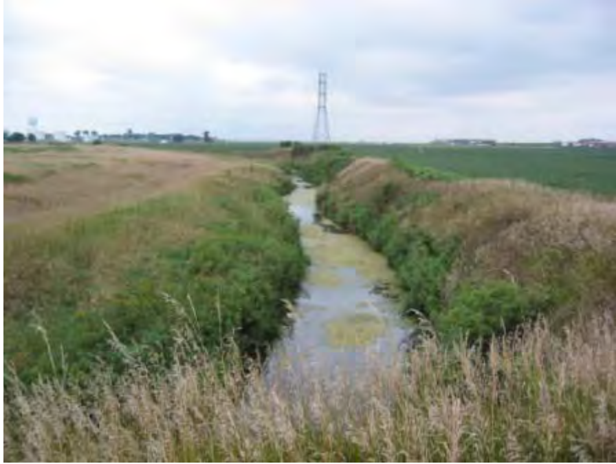
Photo 18. Oak - Air Force Base local drainage looking US from levee road
