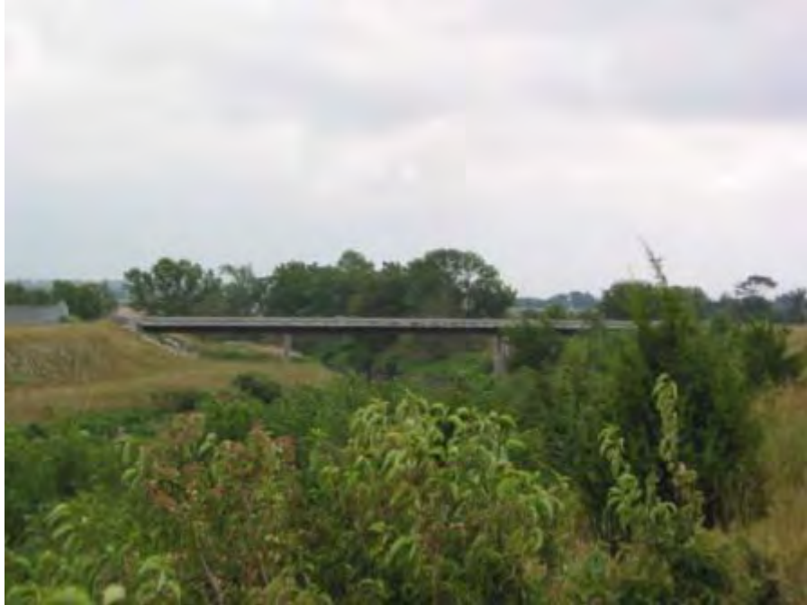
Photo 36. Oak - US face of airport bridge
