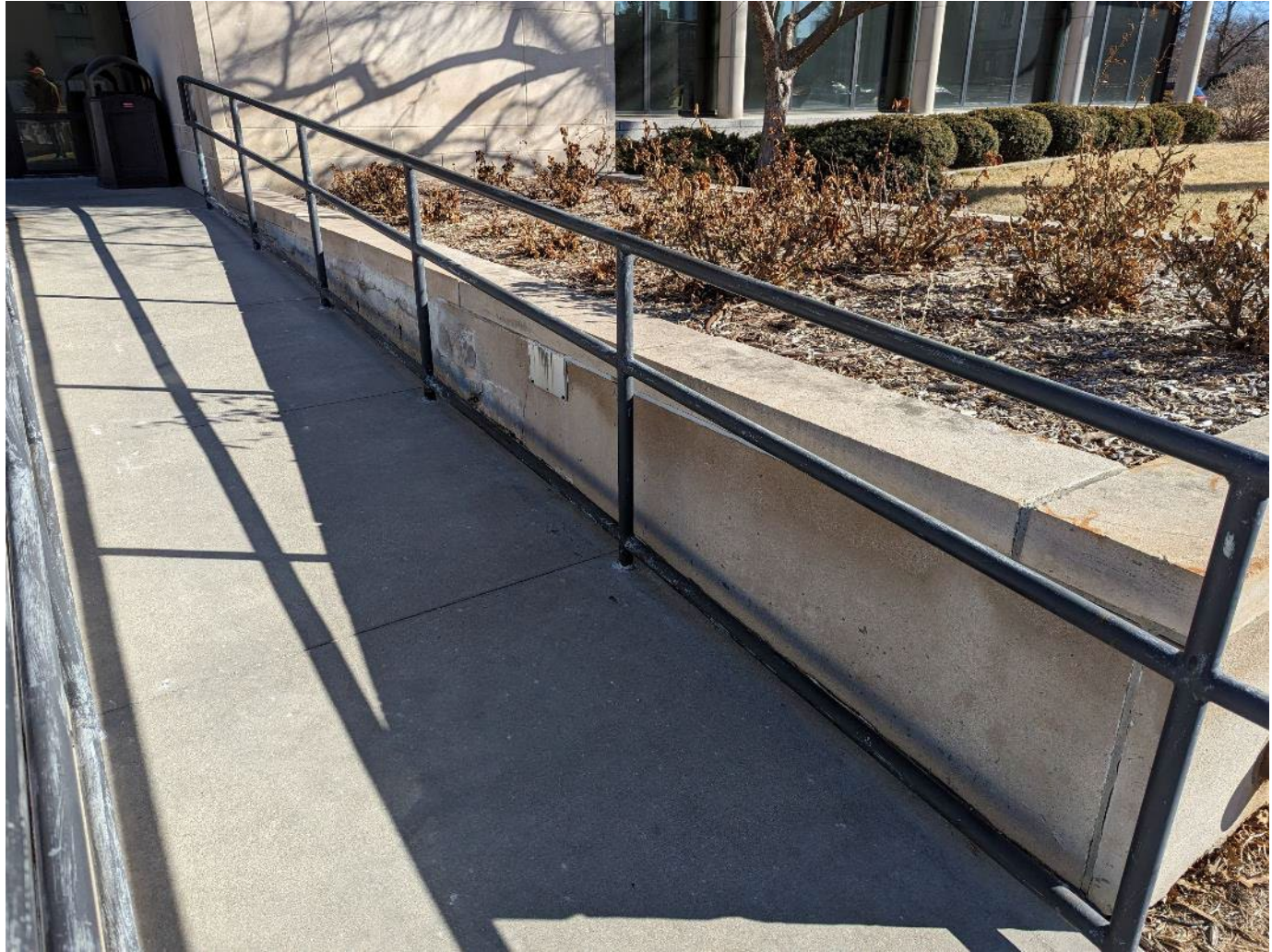
Damaged Limestone Wall and Non-ADA-Compliant Ramp
