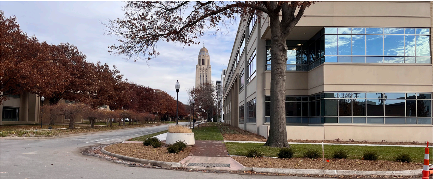
2 Landmark Centre on Lincoln Mall - Complete
