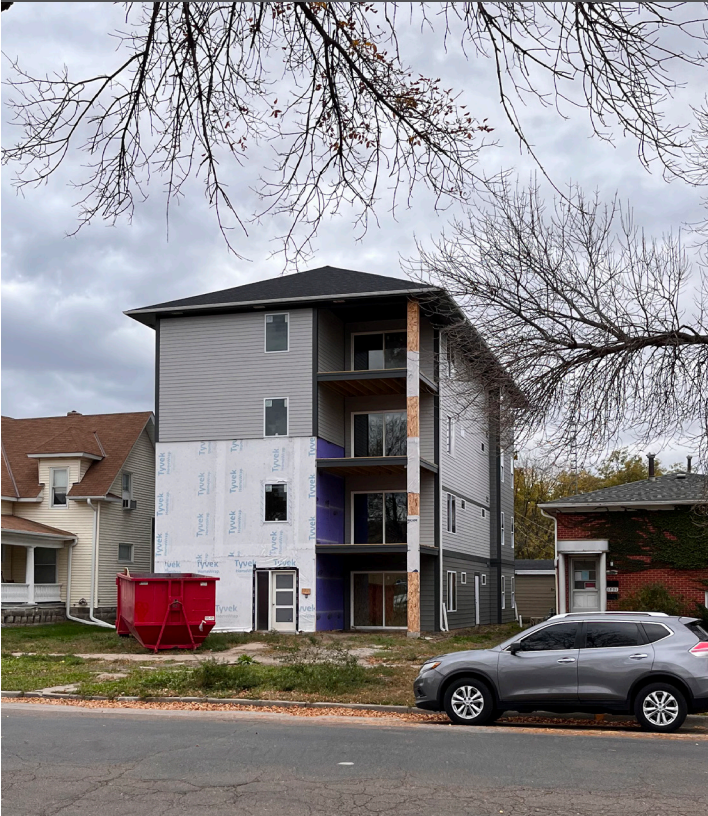
1515 F Street Infill Housing - In Progress
