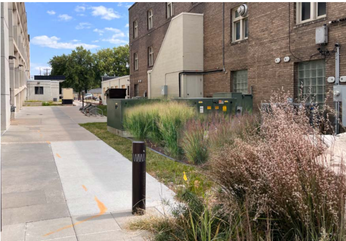
View from Centennial Mall of the existing equipment with the proposed utility box and landscape screening added
