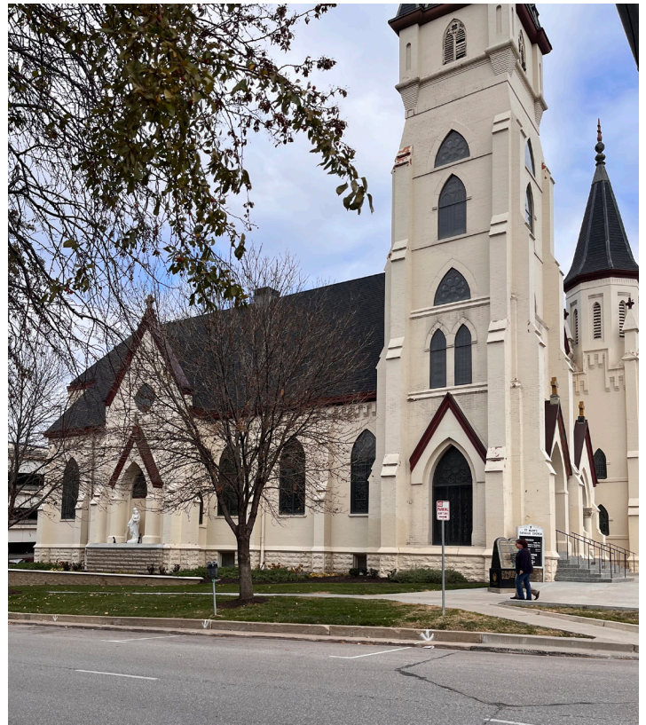
St. Mary's Catholic Church Renovation - Complete
