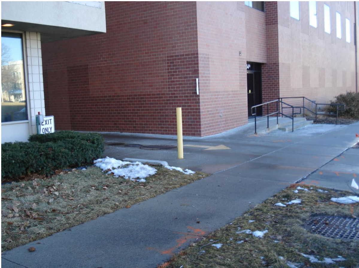
Photo #1: Existing 501 Entry:
