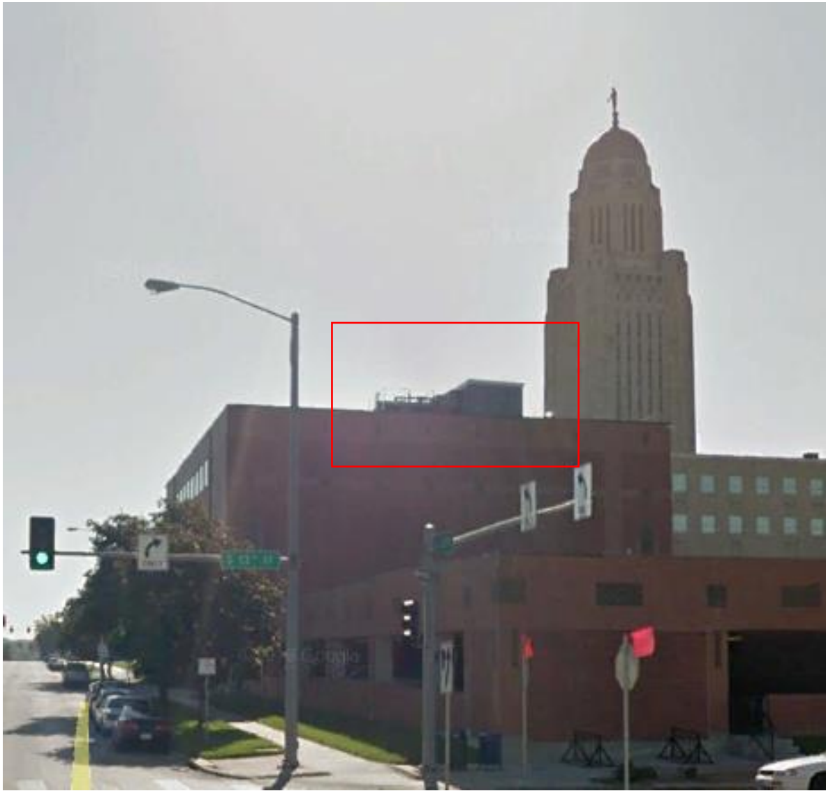
Photo #5: Existing 501 Building as viewed from the 13 th street traffic signal:
