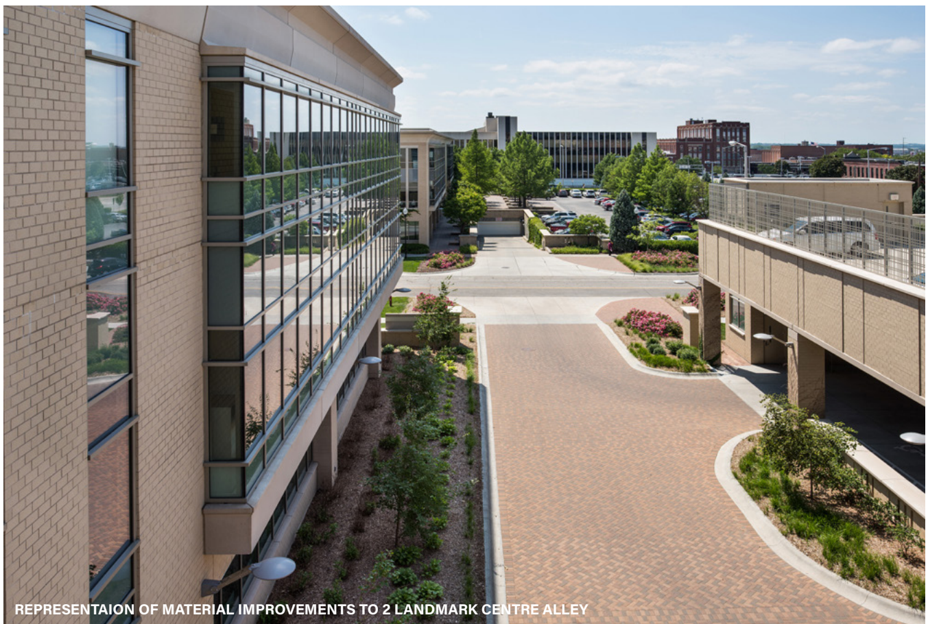
2 LANDMARK CENTRE ALLEY WILL REMAIN OPEN
