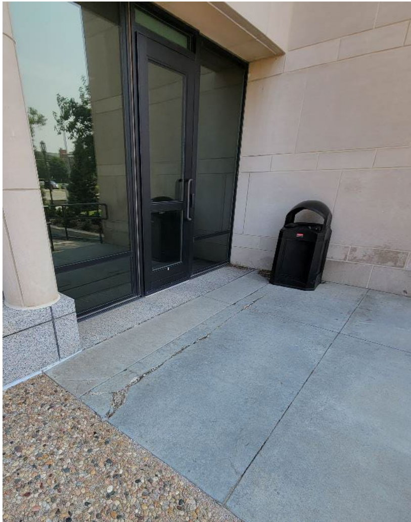
Damaged Granite Walkway & Non-ADA-Compliant Aggregate Surface
