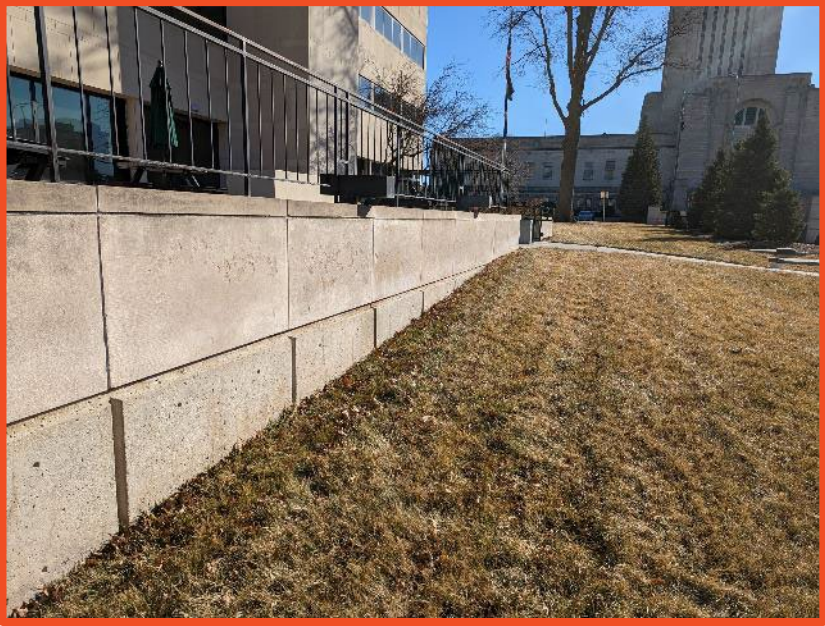
Existing cast-in-place concrete walls with reveals on project
