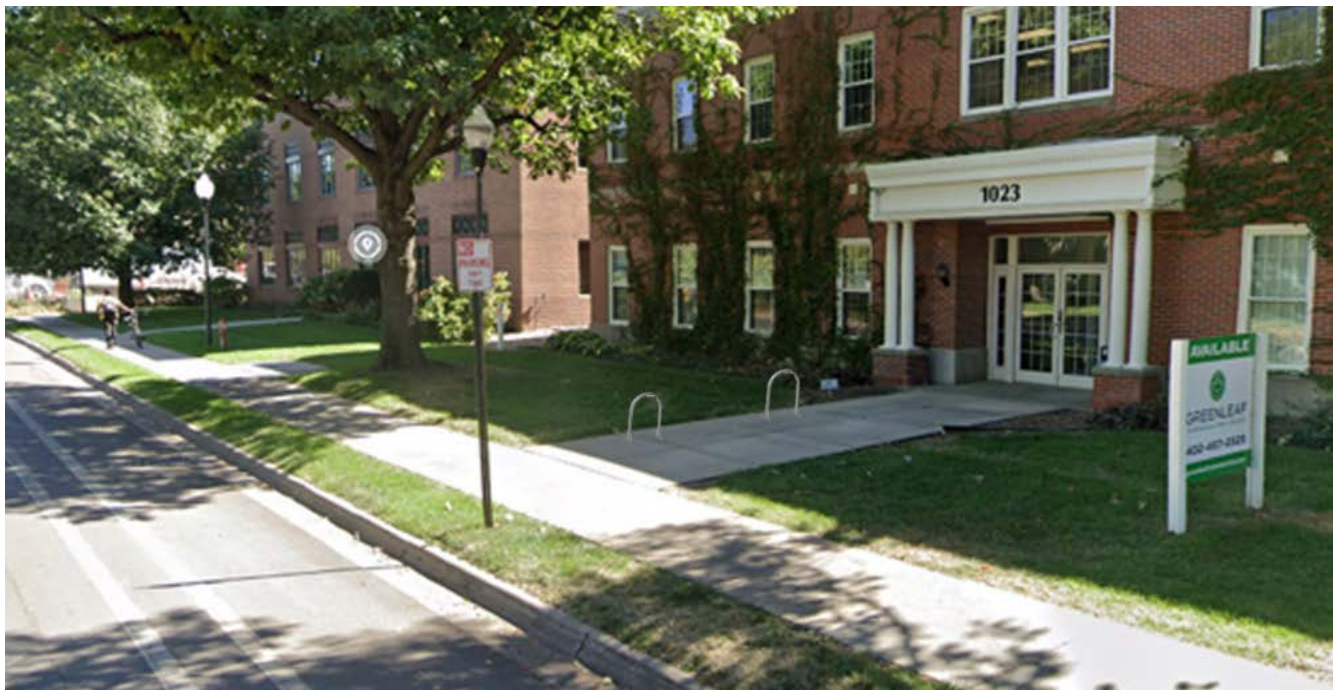
View of two racks placed in front of building
