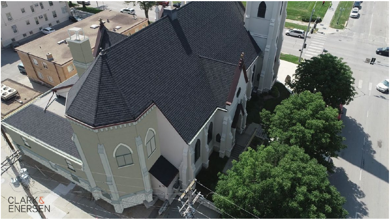
View of the north facade
