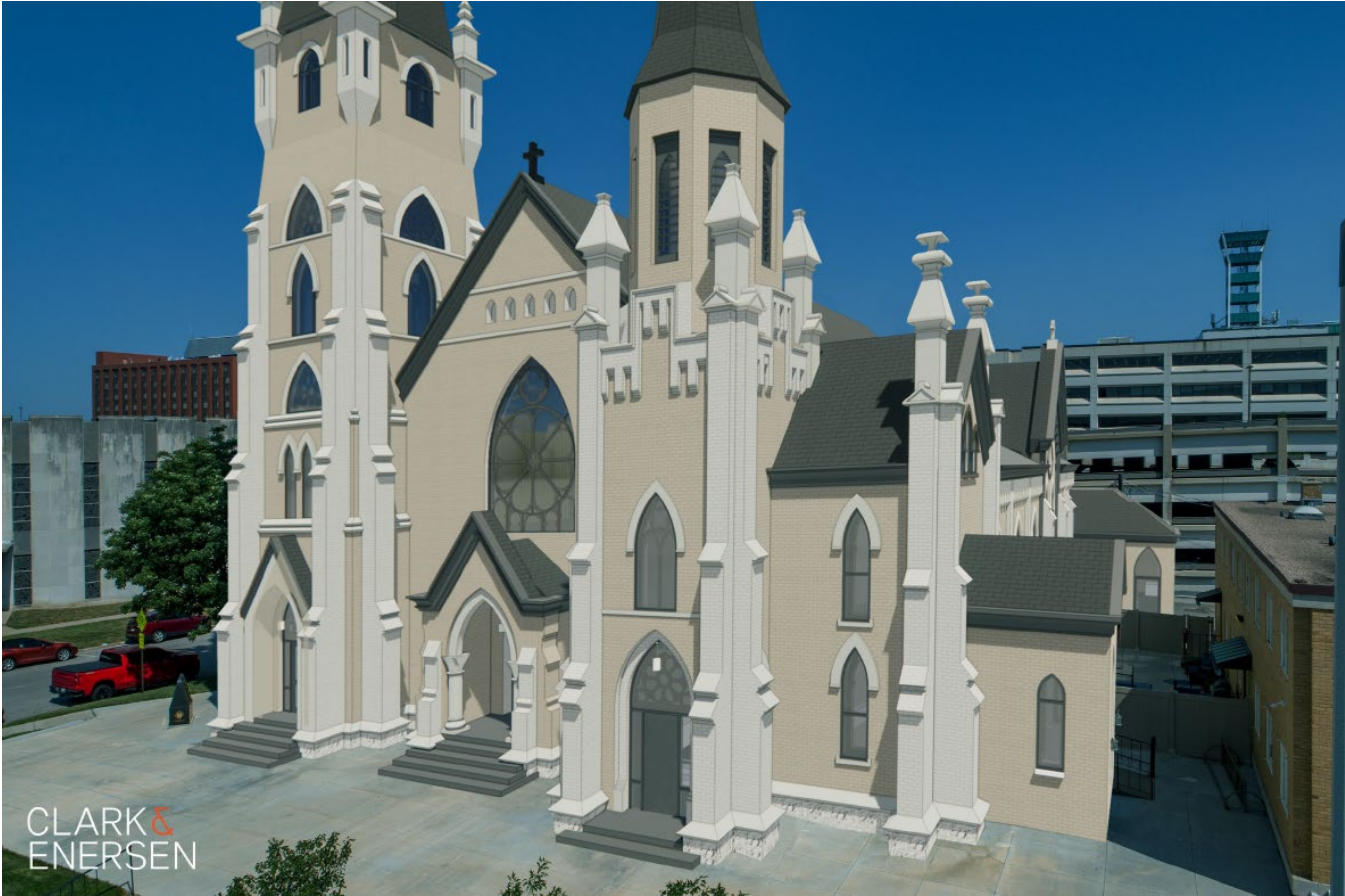
View of the south façade
