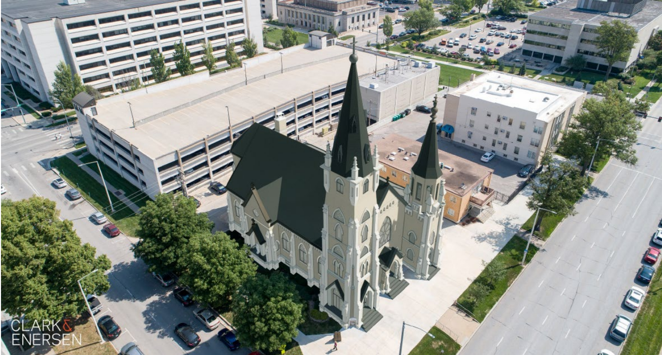
View of the south and west facades
