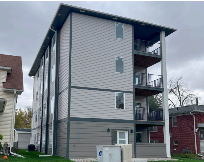
In-Fill Four-Plex (1515 F Street) - In-Progress
