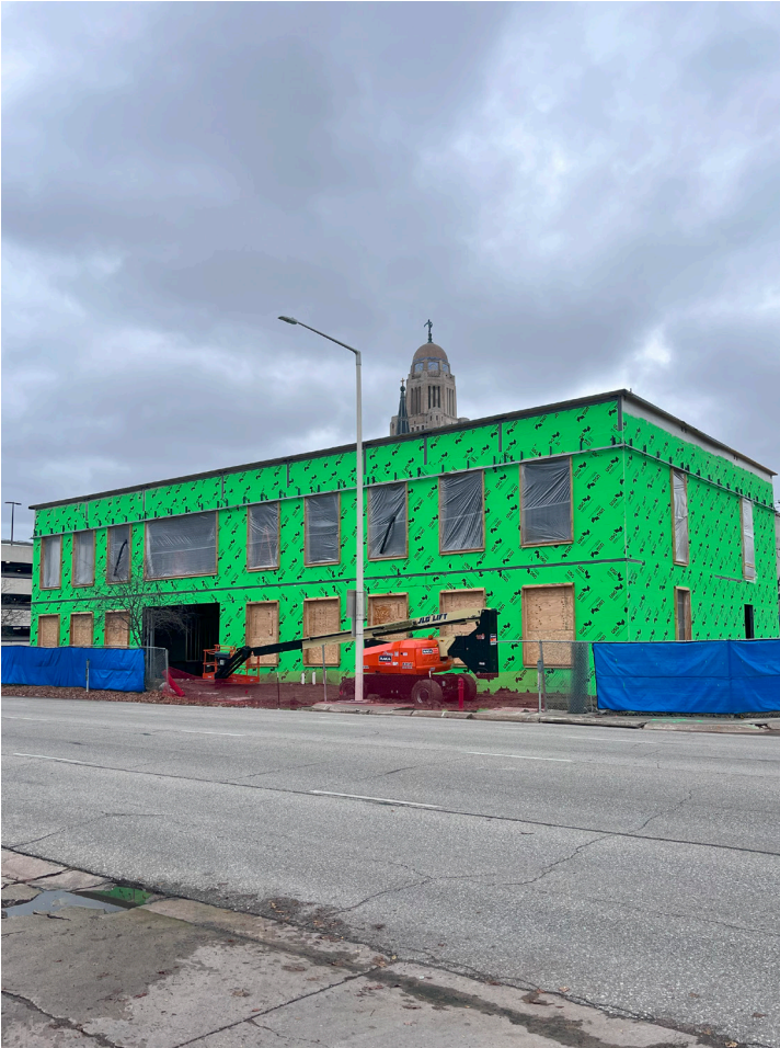
LoNM (1341 L Street) - In-Progress
