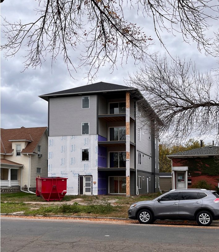
1515 F Street Infill Housing - In Progress
