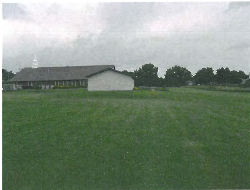
Site Photograph 1 – Looking north at the Property
