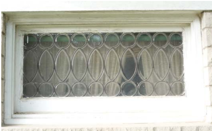
South window of living room
