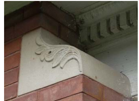
Detail of west chimney
