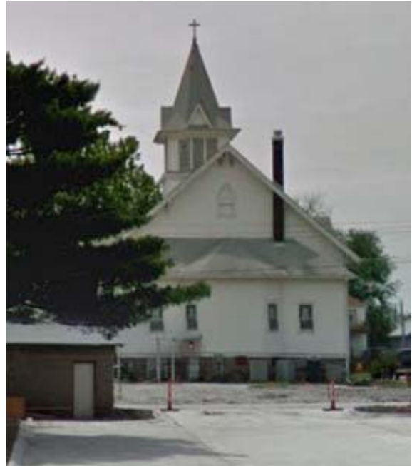
View from north of rear of church
