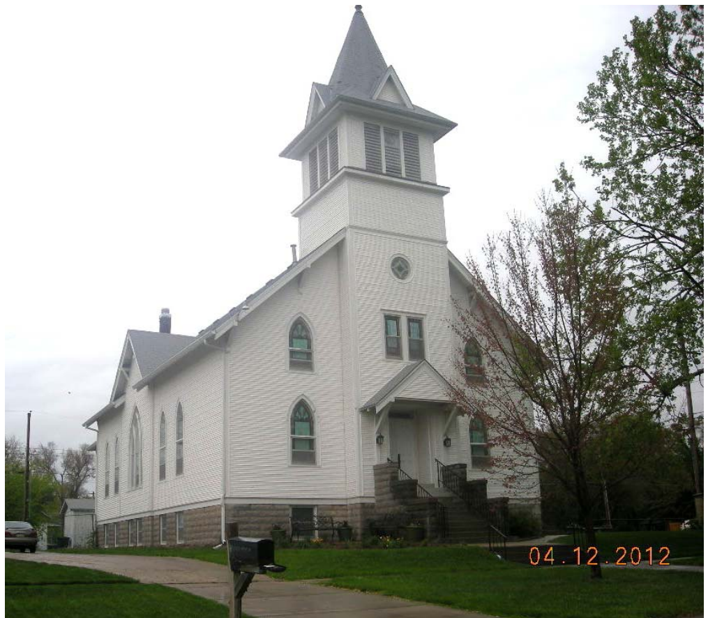
View from south-southwest of front of church
