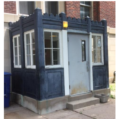
Vestibule at west entrance to Nurses Home/Trabert Hall.
