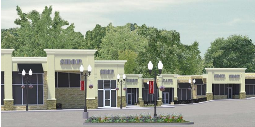
View from Cotner Blvd Looking West
