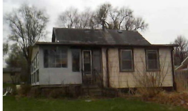
Existing House to be Demolished
