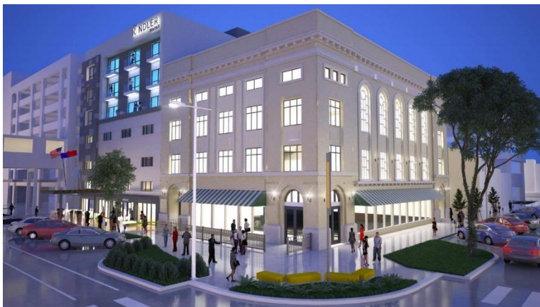
▲ 11 th & P Redevelopment
