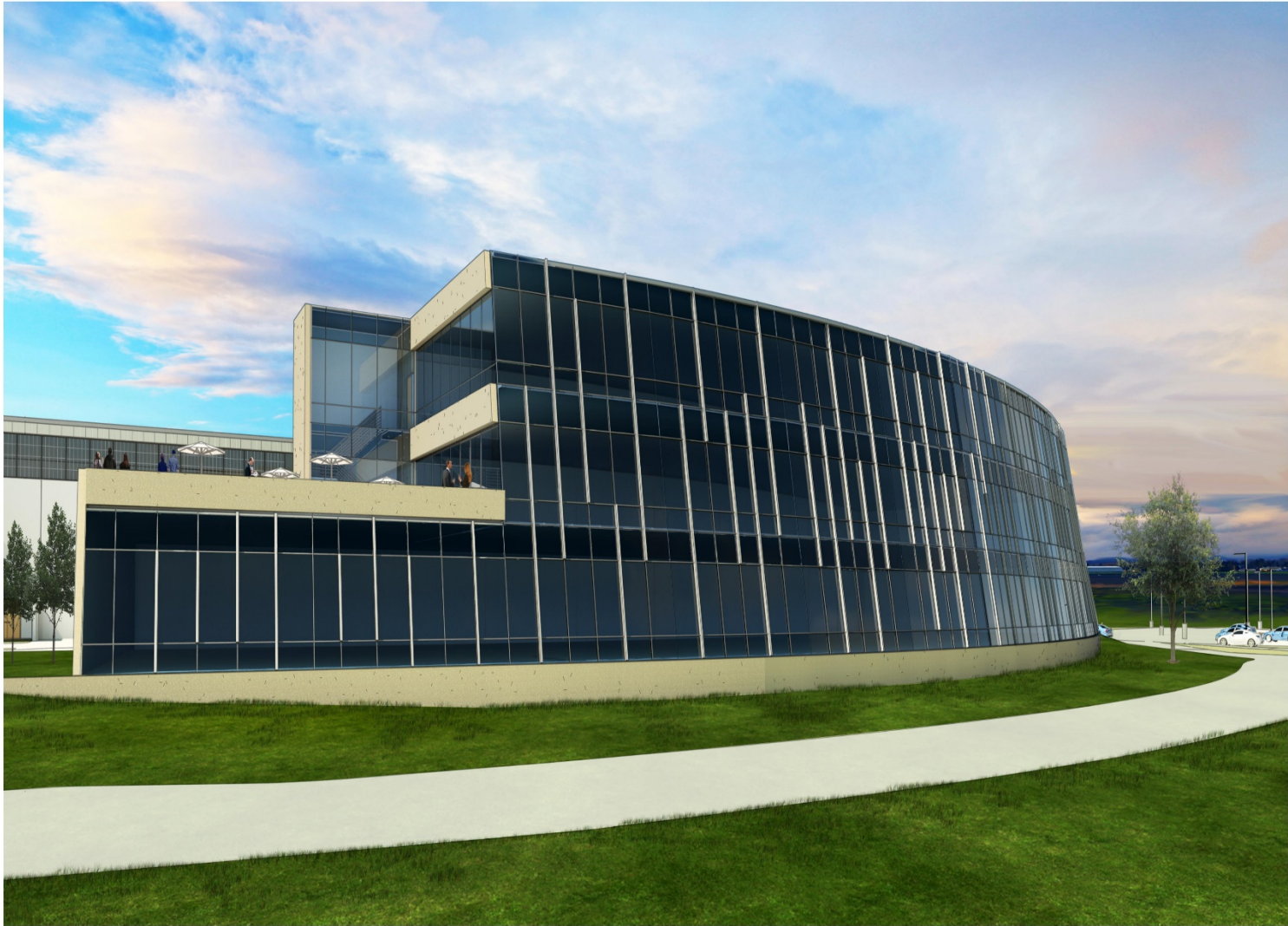
LES Operations Center Office Building – View from the Northeast
