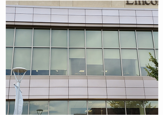
LPS 58th and O METAL PANELS AND GLAZING
