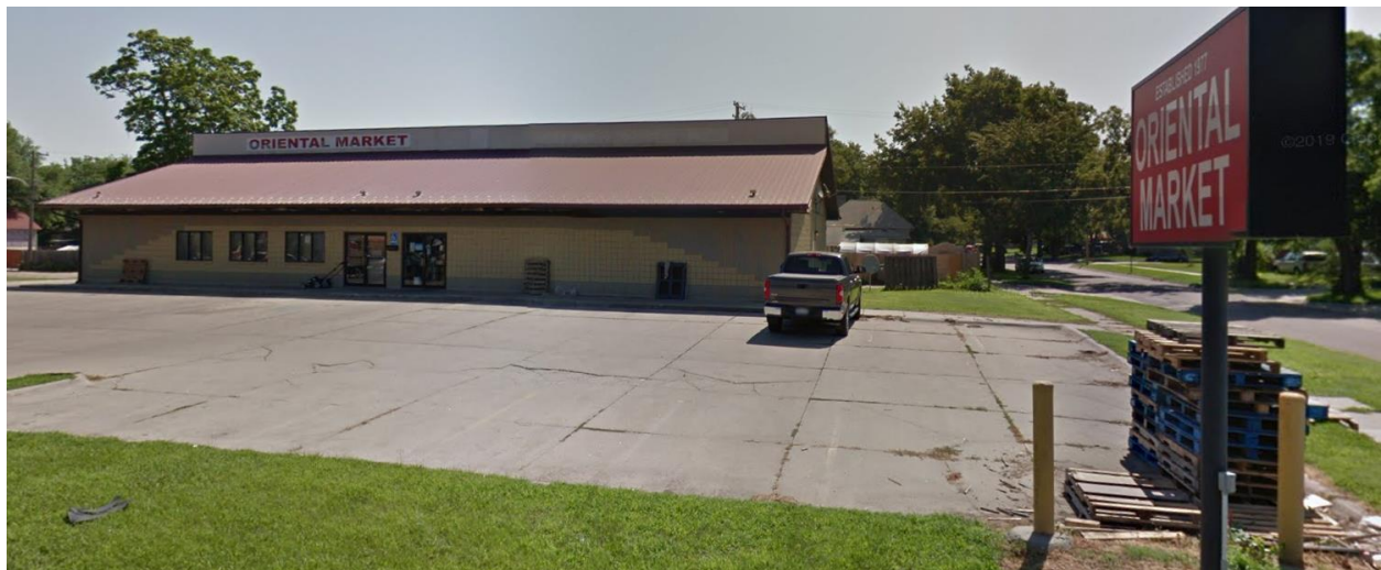
Existing Oriental Market Building
