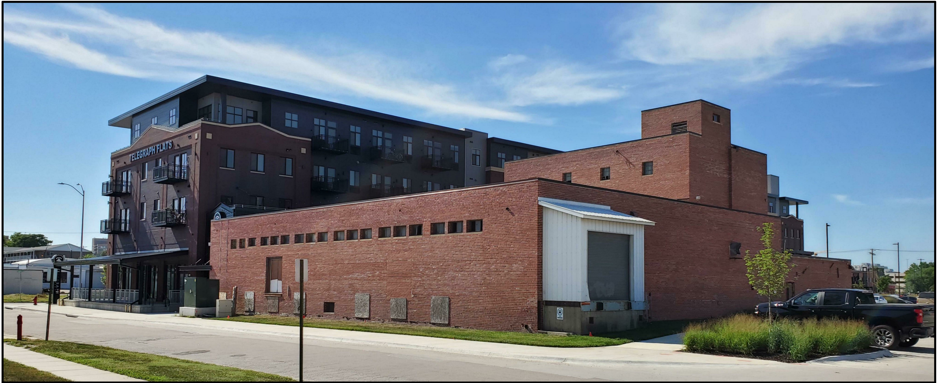
TELEGRAPH WAREHOUSE EXISTING CONDITION
